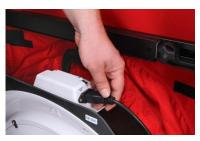
Next, the fan speed controller is connected to the fan and to the power supply.
