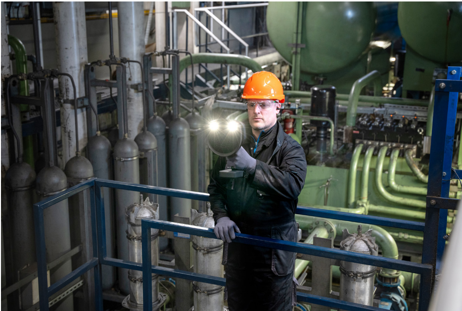
FLIR Si-Series acoustic imaging cameras include features such as dual-mode LED worklights and a 12 MP camera with 8x digital zoom.
